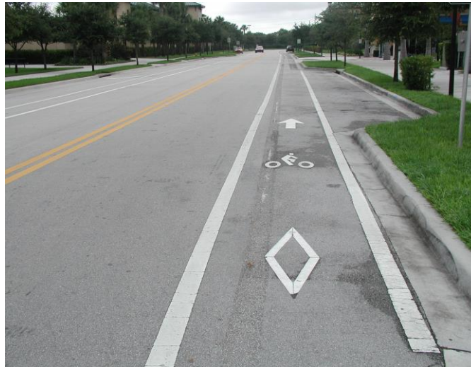
Install bike lanes as wide outside lanes as shown above or as a separate facility
