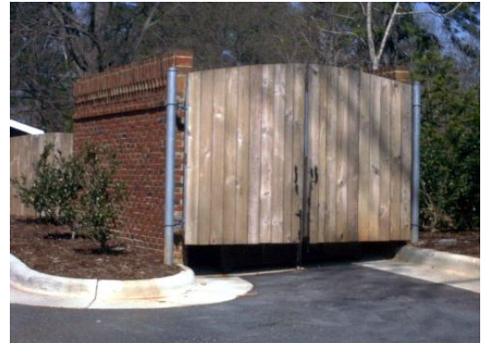
A properly screened dumpster using durable materials matching the principal building
