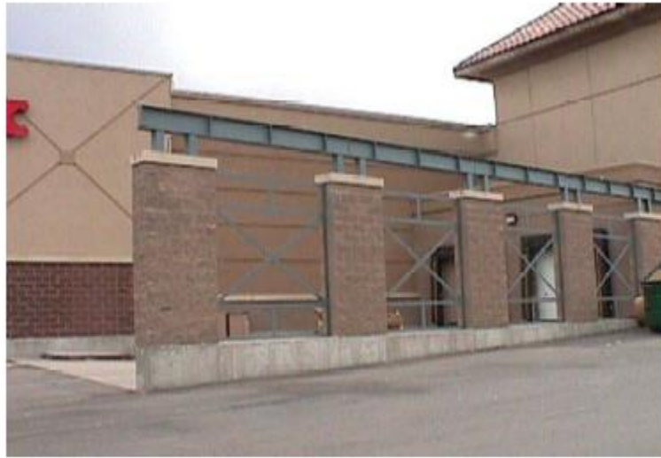
Example of the semi-translucent wall screening used to screen loading dock.
