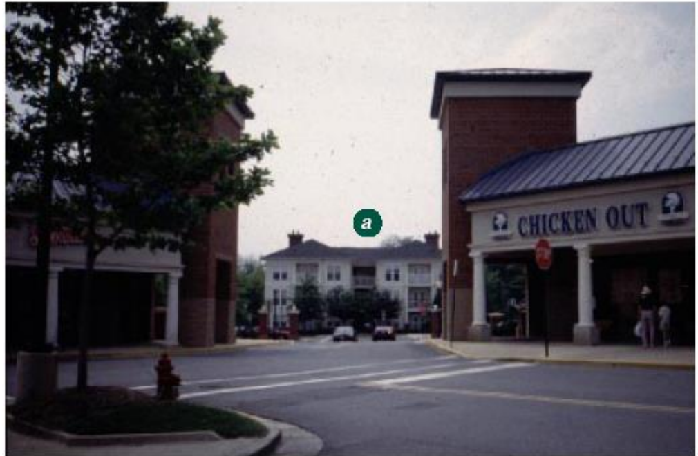
Visual and physical connections are made between this shopping center and the neighboring residential development (a) in the distance.
